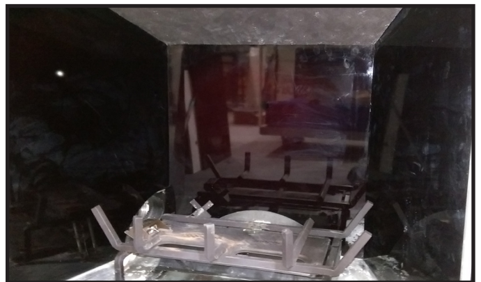
Figure 12 Glass Panels Fully Installed
