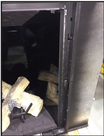
Figure 19 Bracket Installed
